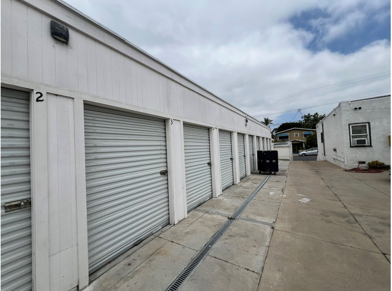
Overview of driveway and garage area (camera facing north)
