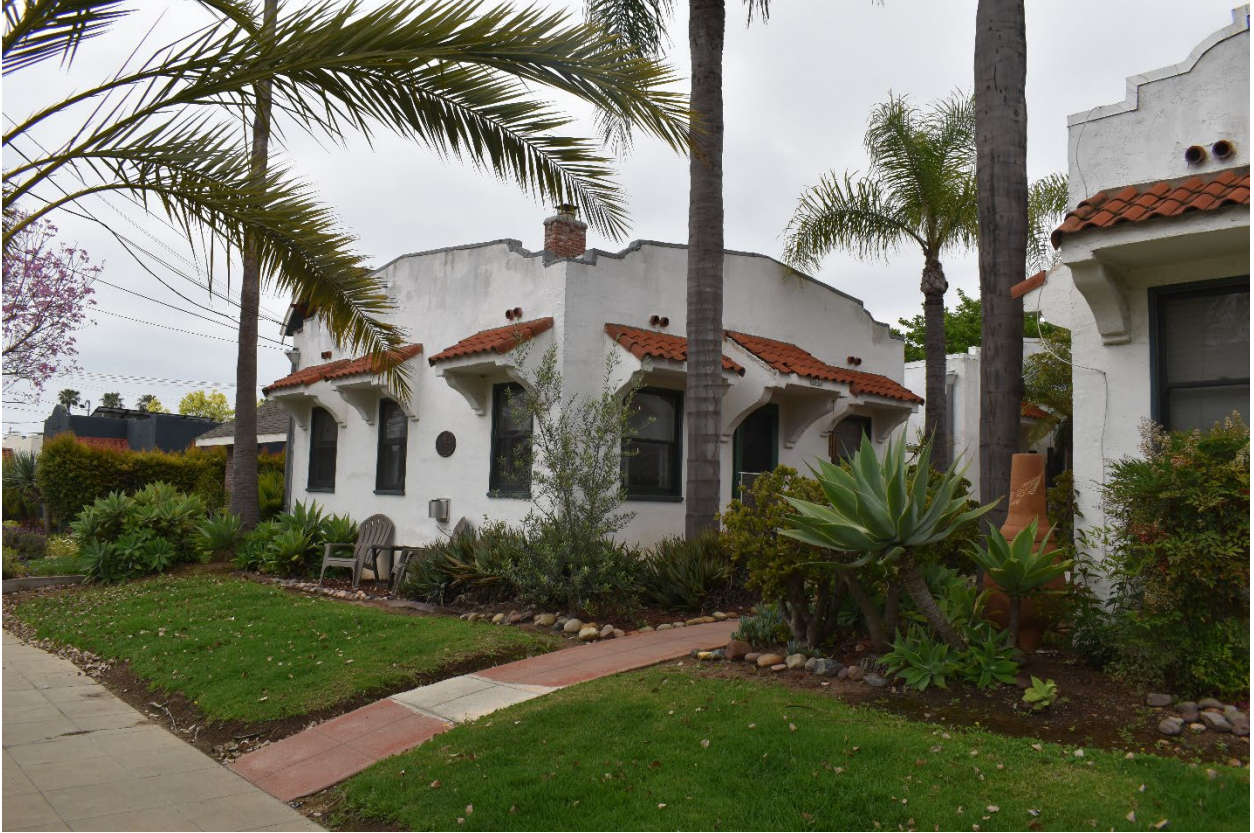
Overview of east and north elevations of detached bungalow located at southeastern corner of property (camera facing southwest)
