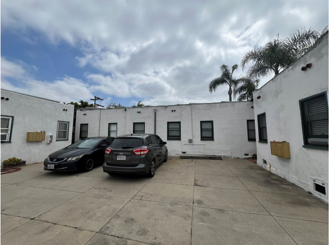
Overview of driveway/parking area (camera facing east)
