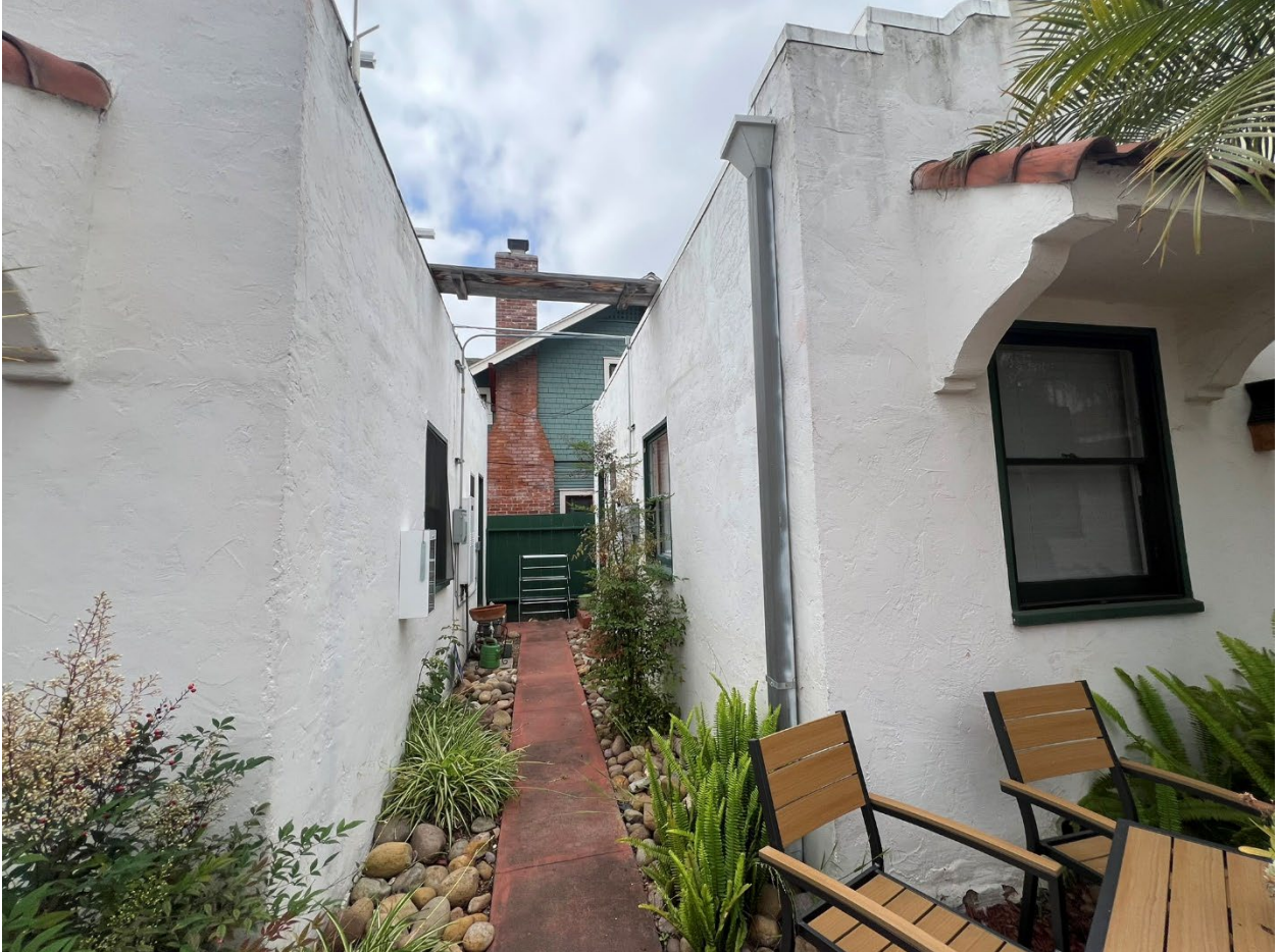
Overview of walkway between detached bungalows along southern property line showing east and west elevations (camera facing south)
