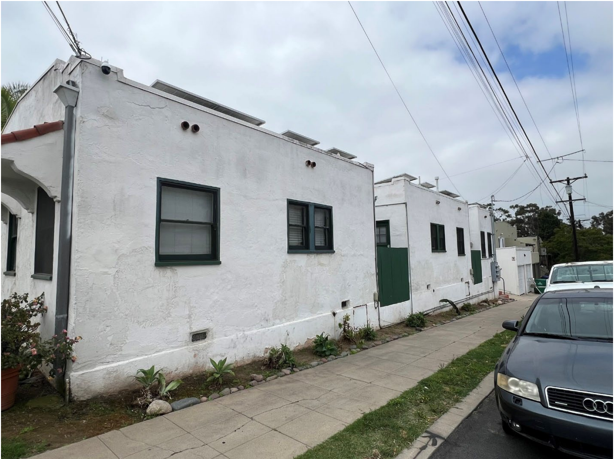
Overview of north elevation of detached bungalows, fronting Elm Street (camera facing southwest)
