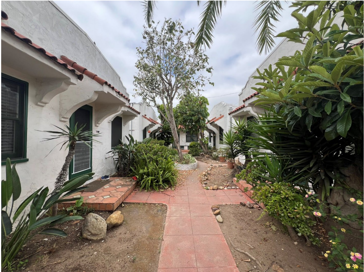
Overview of northern courtyard area with all three types of bungalows framing it (camera facing west).
