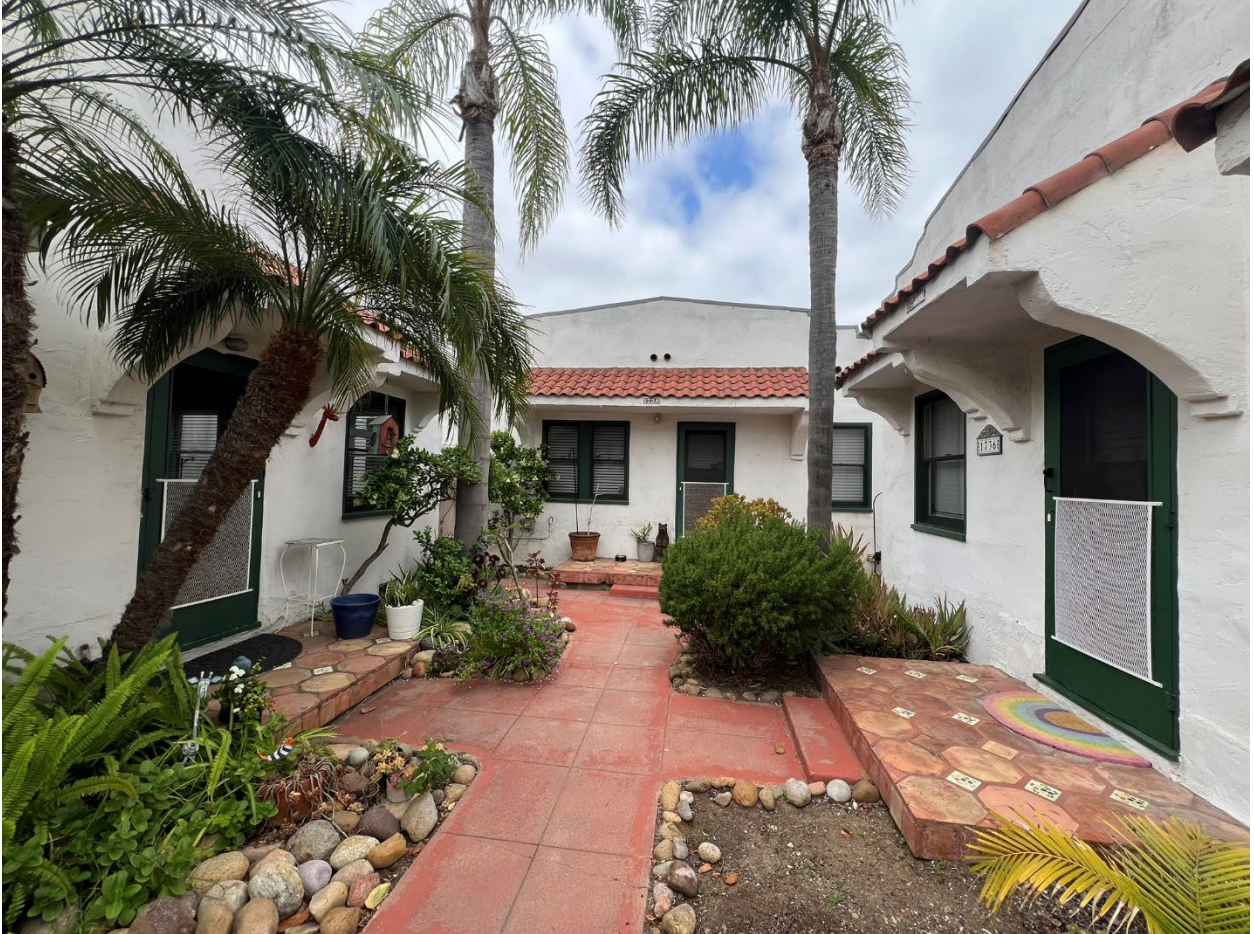
Overview of east elevation of detached bungalow, and the south elevation of the semi-detached bungalow (right) and the north elevation of the detached bungalow (left) (camera facing west).
